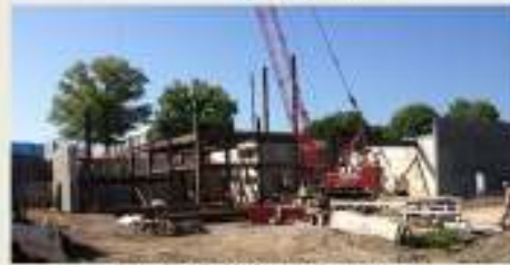
Figure 2: Foundation Steel – Courtesy of Owner
